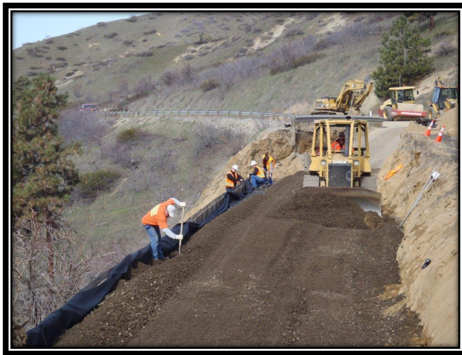
Chelan County Road Crew building an MSE wall on North Dryden Road near Dryden. The project’s goal was to stabilize a chronically unstable roadway embankment.
