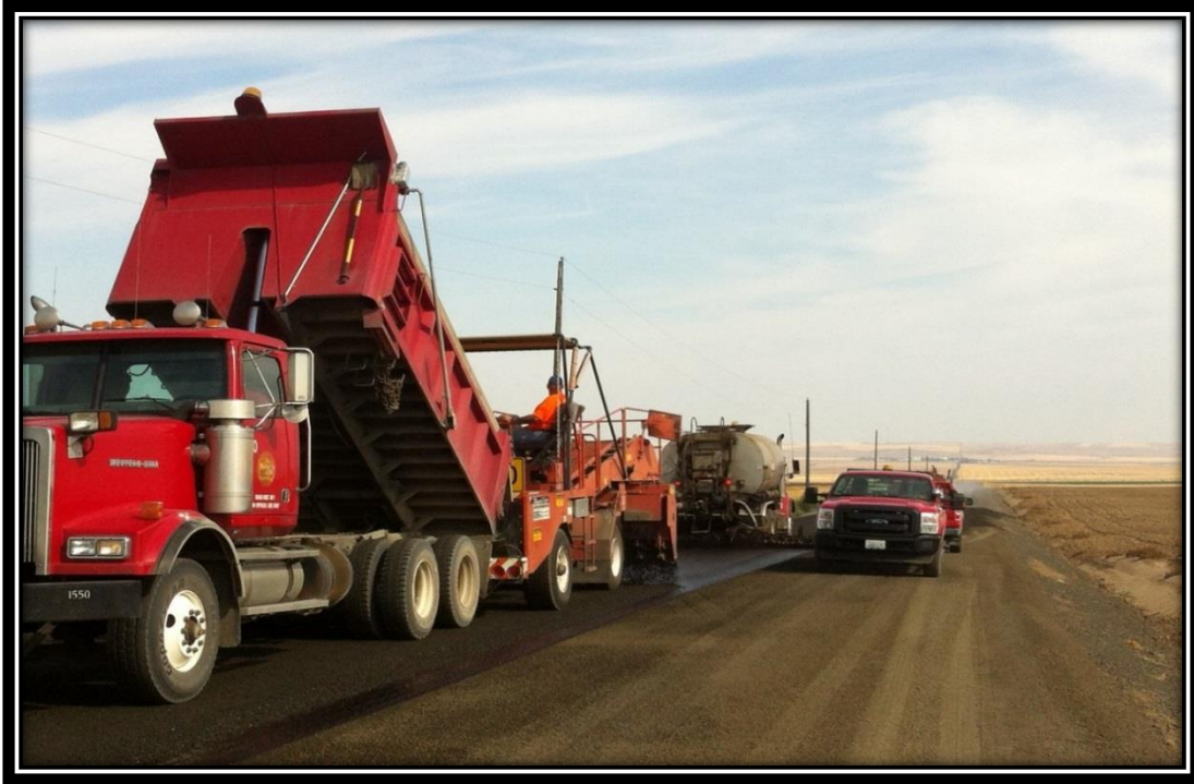
Grant County Road Crew shooting the prime or penetration shot of HFE-150 on the last phase of R-NE between Wilson Creek and Hartline.
