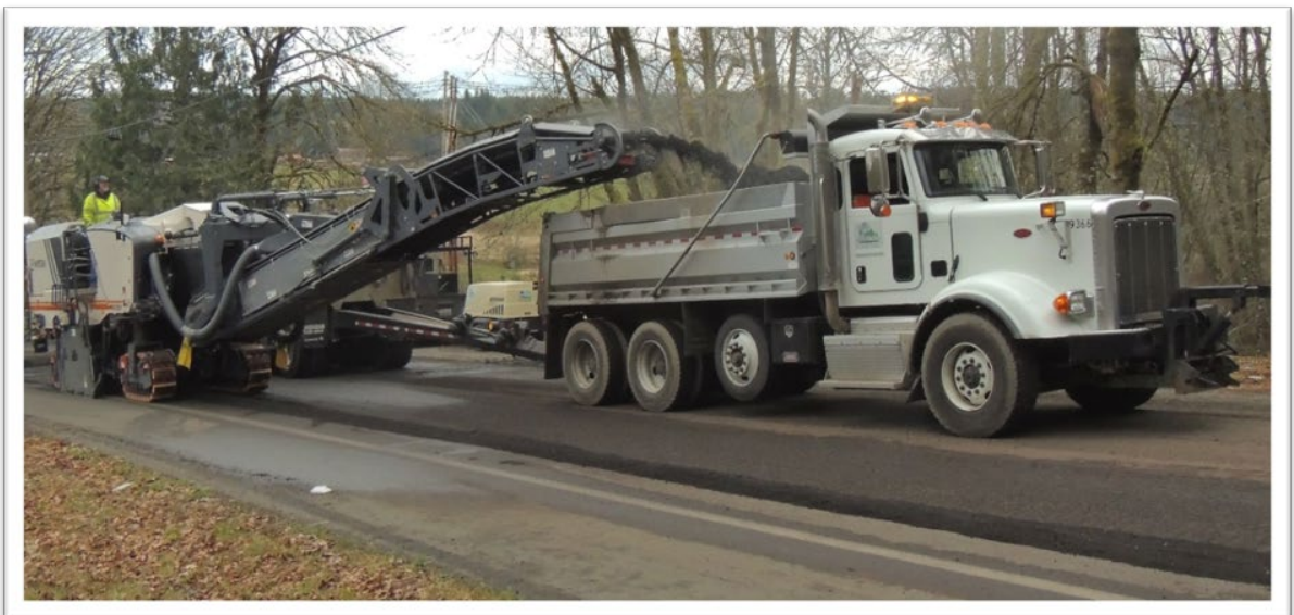
Photo –Thurston County Public Works ( asphalt cold milling process )
