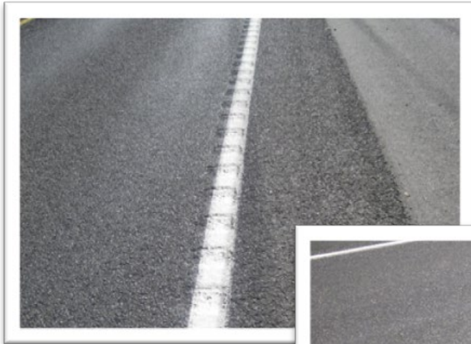
Recessed shoulder rumble strips
