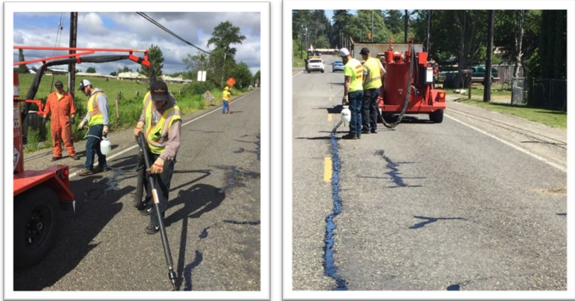
Photo –Grays Harbor County Public Works ( Crack Sealing )
