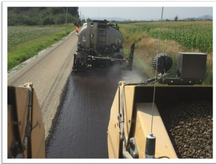
Photos–Skagit County Public Works ( Chip seal and wheel path application )
