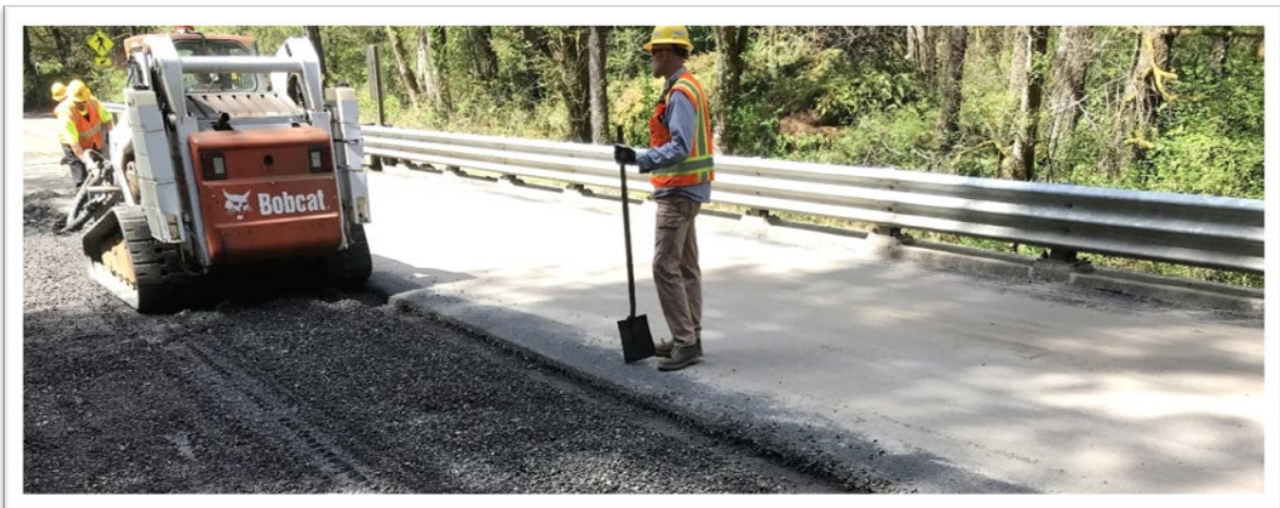
Photo - Clark County Public Works ( Milling )
