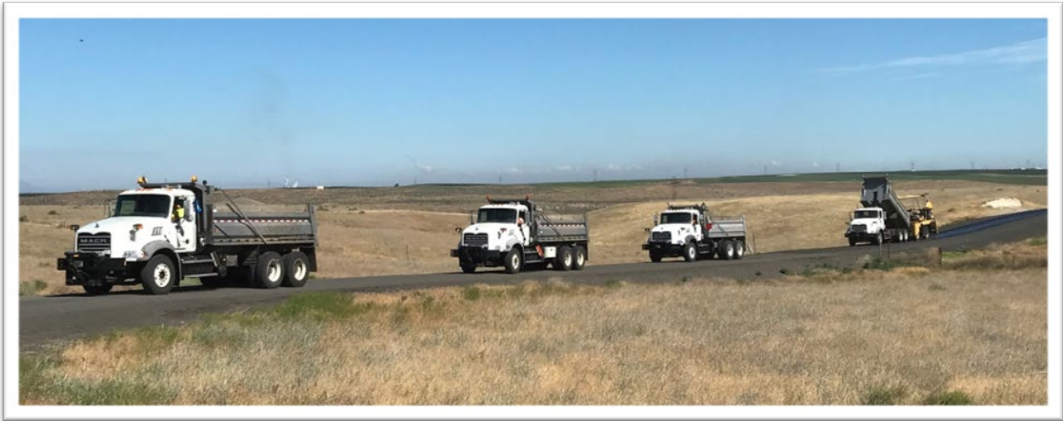
Photo – Walla Walla County Public Works ( Chip Sealing )
