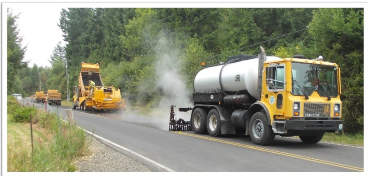
Photo – Cowlitz County Public Works ( Chip Sealing )
